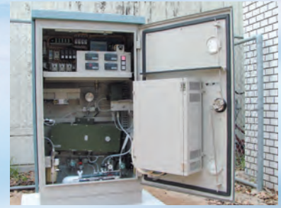
水質監視装置 Water Quality Monitoring Equipment
