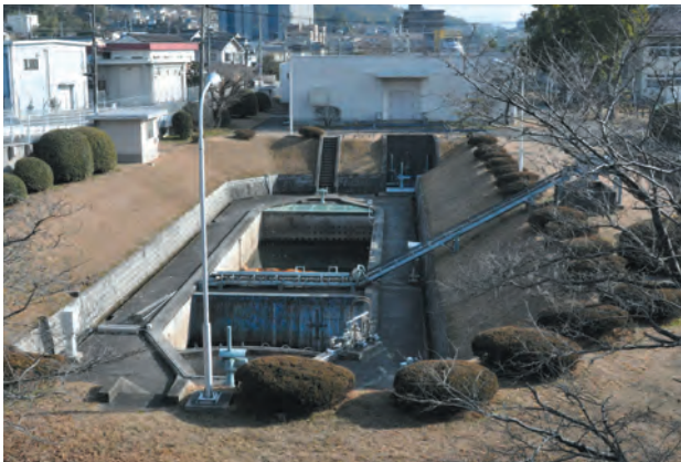
戸坂取水場 Hesaka Intake Station
