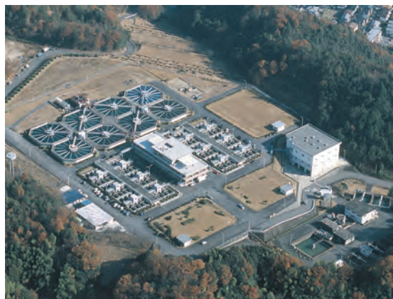
緑井浄水場 Midorii Purification Plant
