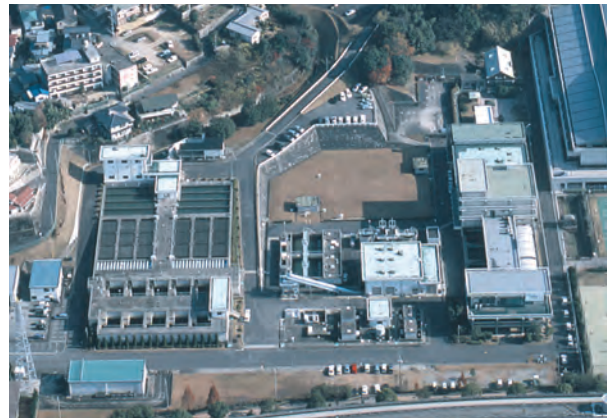
牛田浄水場 Ushita Purification Plant
