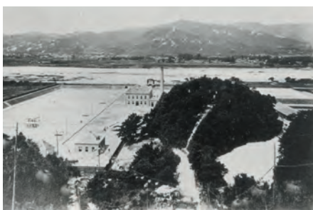
創設当時の緩速ろ過池(1898~1984) Slow sand filters right after construction (1898-1984)
